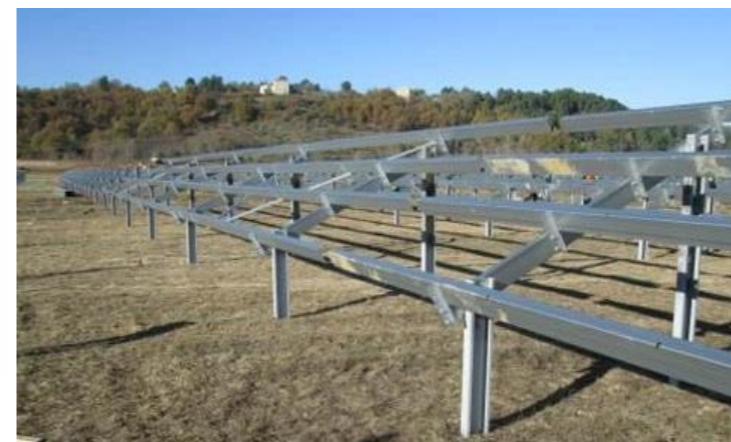
Figure 5 : Structure porteuse (2 ancrages pieux)
